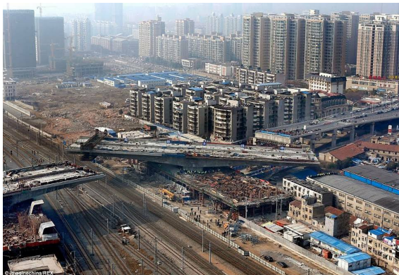
ചിത്രം 20: Rotating the bridge deck to align with the existing road.
