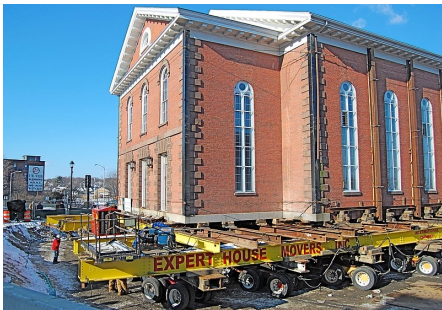
ചിത്രം 6: Hydraulically powered dollies move a historic 19th-century brick church in Salem, Massachusetts. Source: Wikipedia
